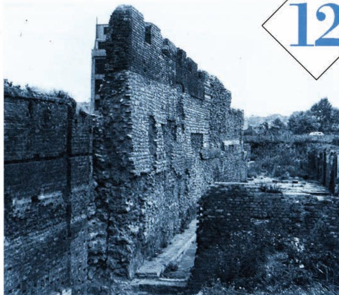
Roman, Medieval and later City Wall in St Alphege churchyard exposed after World War II damage.
